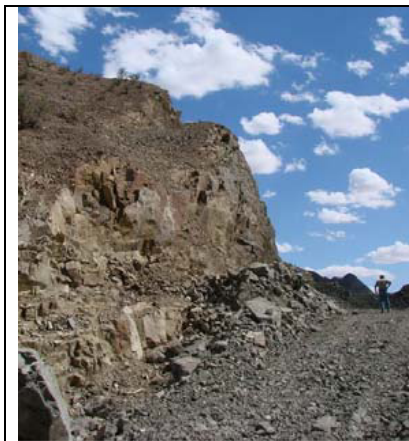
Figure 9. Block fall due to toppling
