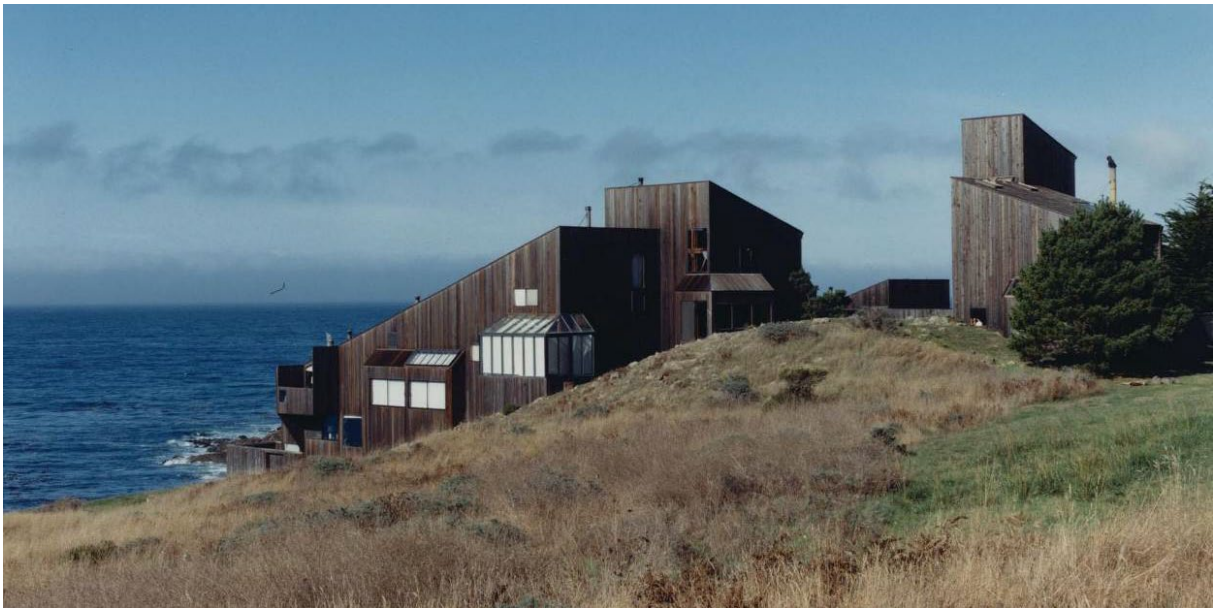
Figura 22. Charles Moore, Donlyn Lyndon, William Turnbull y Richard Whitaker, Sea Ranch Condominium I , 1963, California Foto: MLTW Collection, Environmental Design Archives, University of California, Berkeley
