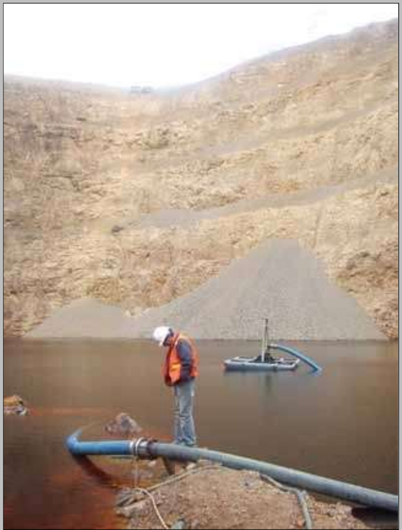
Dewatering collection pits
