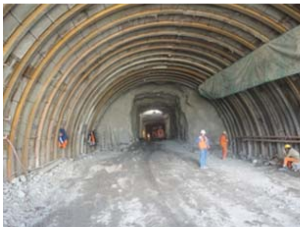
Figure 13. Excavation partition of crown
