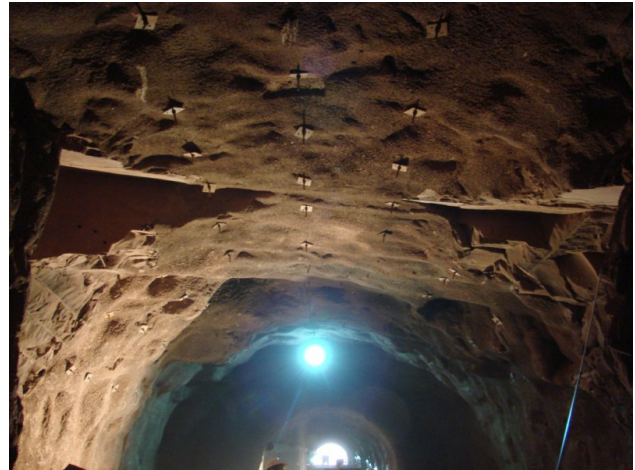
Figure 11. Typical rock wedges formed in T5
