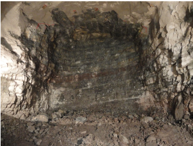
Figure 7. Excavation front within horizontal layers of shale and sandstone in T1.
