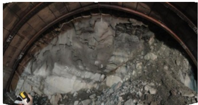
Figure 9. Stepped and rotated blocks in T3.
