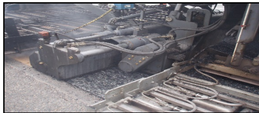
Figure- 6 Scarifying and heating unit
