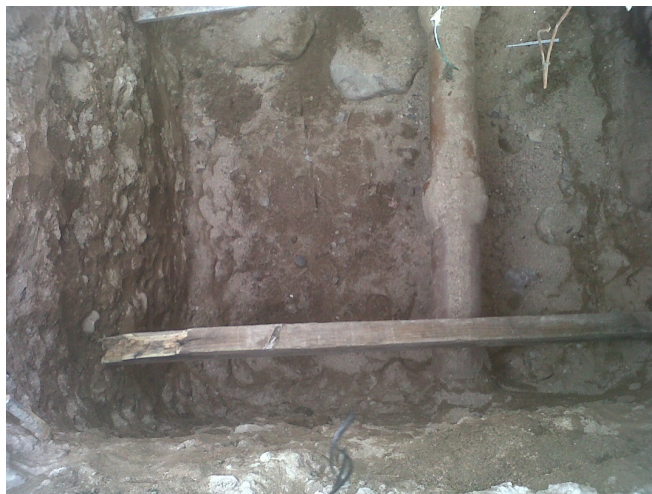
Figura 6.8: Cloaca obsoleta
