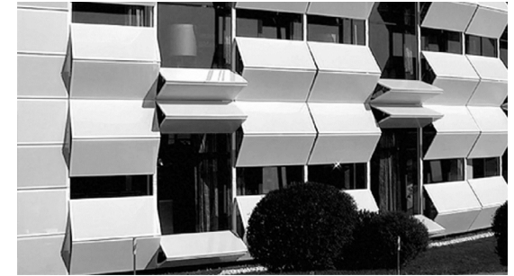
Figura 8. Fachada cinética - Kiefer technic Showroom, Austria, 2007 / E. Giselbrecht+Partner [foto: Paul Ott, en https://architizer.com/projects/showroom-kiefertechnic-architecture/ ]
