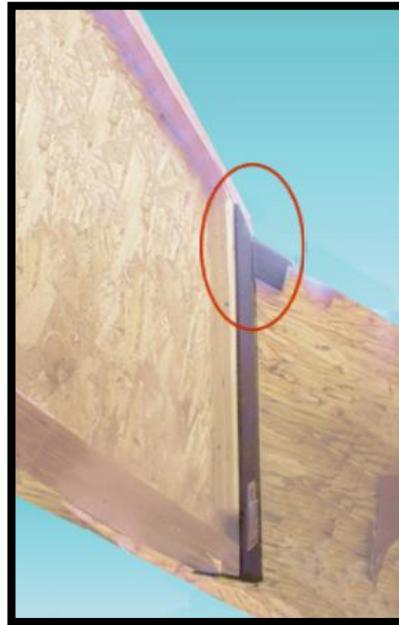
**Figura V-27: Skew and Slope Hanger. Fuente: Hanger Lesson by RedBuilt.**
