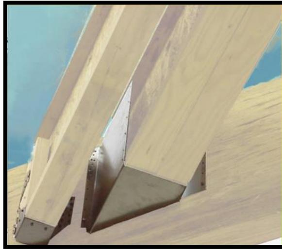
**Figura V-25: Skew Hanger. Fuente: Hanger Lesson by RedBuilt.**
