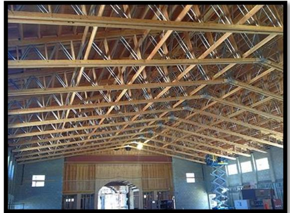
**Figura V-1: Taylor Middle School Cafeteria. I-Joists y Open Web. Fuente: Fuente: RedBuilt Engineered Wood Products.**
