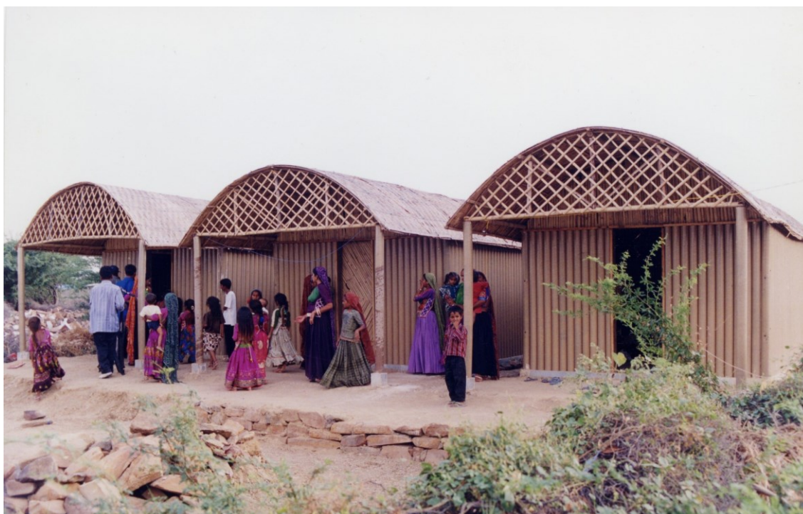
Figura 33. Paper Log House, Bhuj, India, 2001.
