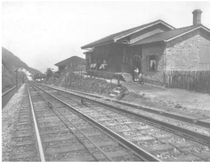
▪ Fig. 5. On the route of a cable-worked mainline railway; the five-section Serra inclines on the São Paulo Railway. Clearly visible are the haulage cables and pulleys, the steepness of the grade, and the workers houses alongside with wives and children, and a wisp of steam in the distance from the winding engine. P Mahoney collection.
