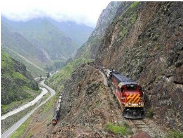
▪ Fig. 1. The Ferrocarril Central in Peru, opened in 1893, showed the world what was possible to make standard gauge and exceptionally steep gradients workable in situations where there was sufficient value of traffic available to cover the unavoidably high operating costs. It likely also demonstrated the shortcomings of such a railway and possibly dissuaded others from copying it. Here modern freight trains traverse three levels of switchbacks in 2013. Credit: Kabelleger, David Gubler, Wikimedia Commons.
