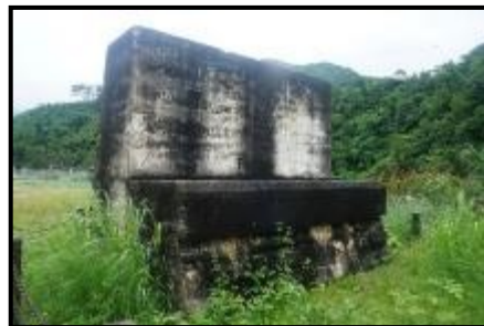
The site of Mangbang bridge along the Burma Railway
