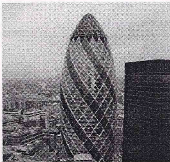
Fig. 5. Swiss Re Headquarters Piel estructural
