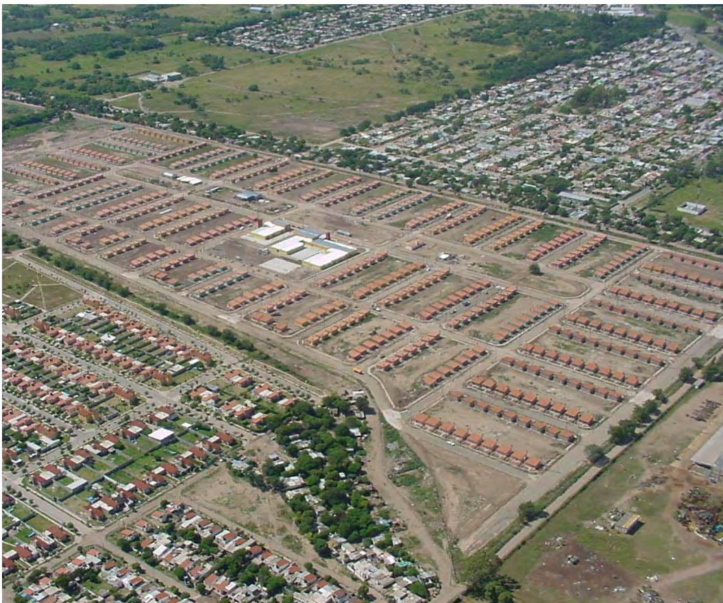
Photo 18: Aerial view of subsidised housing and the urban context
