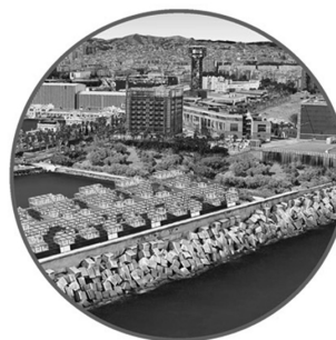
Expanded city: over infrastructures
